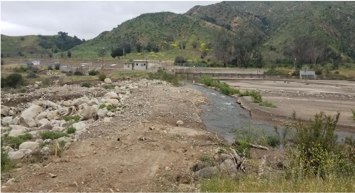
Photograph 3 View standing on the east side of the timber cut-off wall, downstream of the Forebay area, looking west toward the Facility. The Robles Facility cannot operate if the timber cutoff wall is breached because no forebay can be maintained. At this time, the volume of sediment in the Forebay that was deposited during storm events will need to be removed to enable the Facility to operate as designed, both for water diversions and safe fish passage (April 16, 2019).
